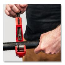
1. Cut pipe square using a fine-toothed saw or displacement-type metal tubing cutter.
